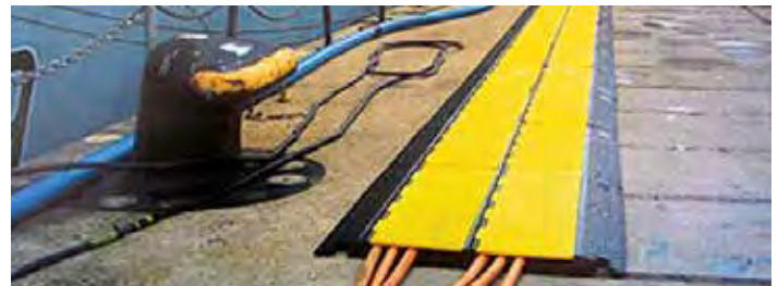
AMS® in use at Naval dock yard
